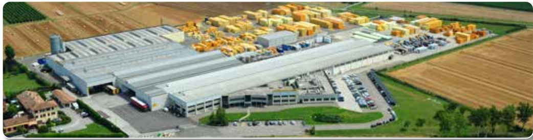
HEADQUARTERS DUNA-CORRADINI Spa (Soliera - Italy)
